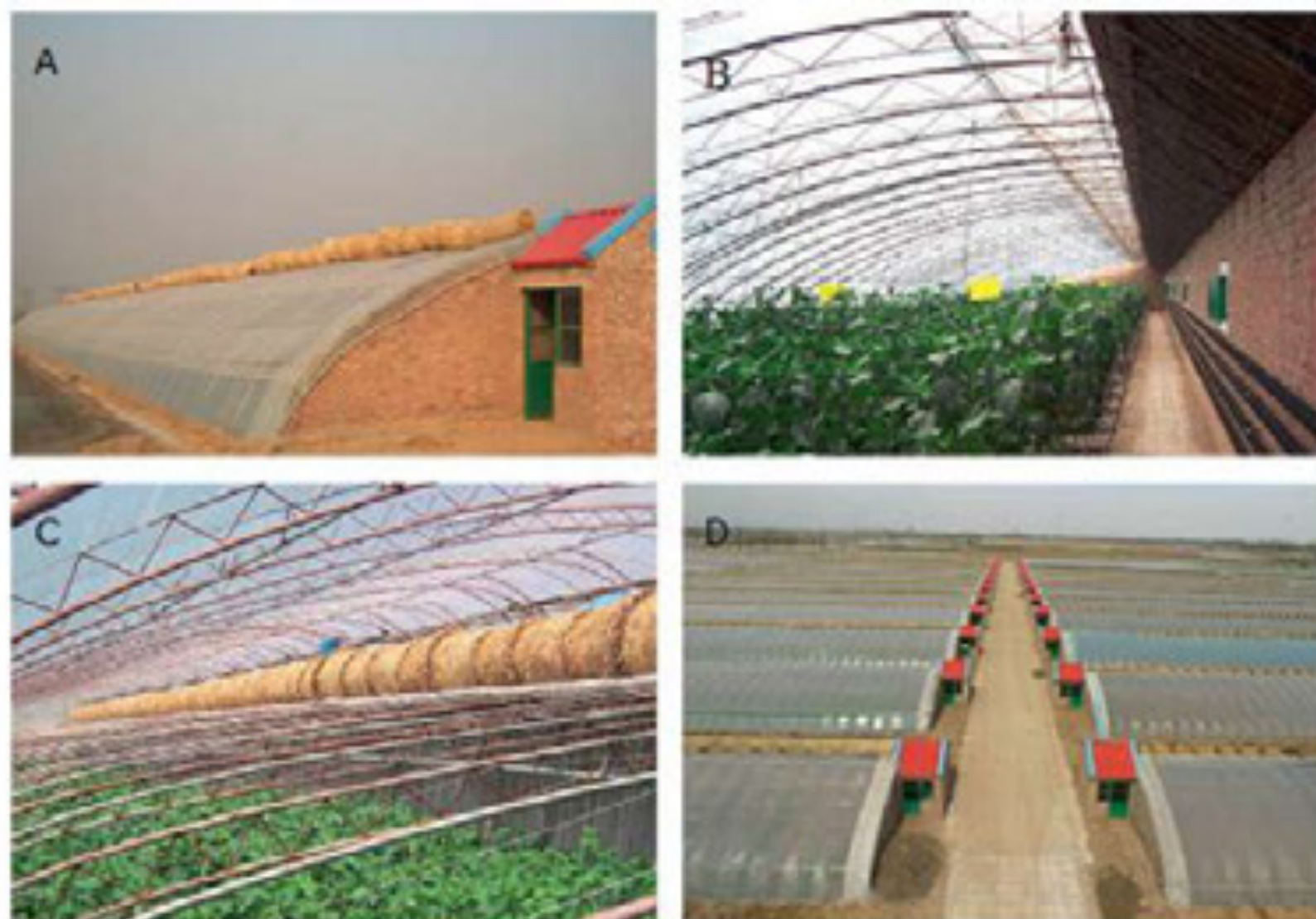
Fig. 2. Photos of a single-slope solar greenhouse: (A) exterior, (B) interior, (C) upper side of the double-arch solar greenhouse, and (D) a group of solar greenhouses. (Photos A through C were provided by M. Qu and Z. Zhang, respectively; photo D is courtesy of Beijing Agricultural Bureau).
